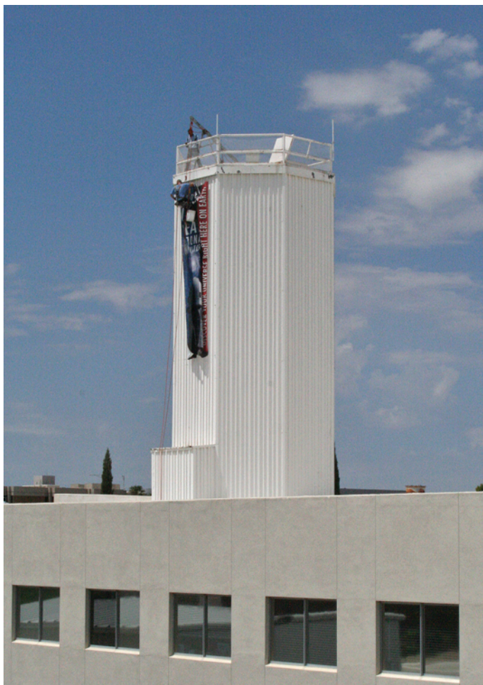
Installing the banners. (Image credit: Pete Marenfeld/NOAO/AURA/NSF.)
